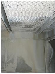
Regular inspection, monitoring and tests were carried out over several months. These showed that not only had the technology prevented the build-up of scale in the recirculating system, but also removed existing scale which had formed in pipework despite the water softening equipment.
